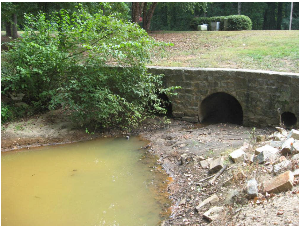
PHOTO – QQQ: downstream face of Shirley Bridge Road culvert; sediment has settled out where channel has been widened in the vicinity of the culvert
