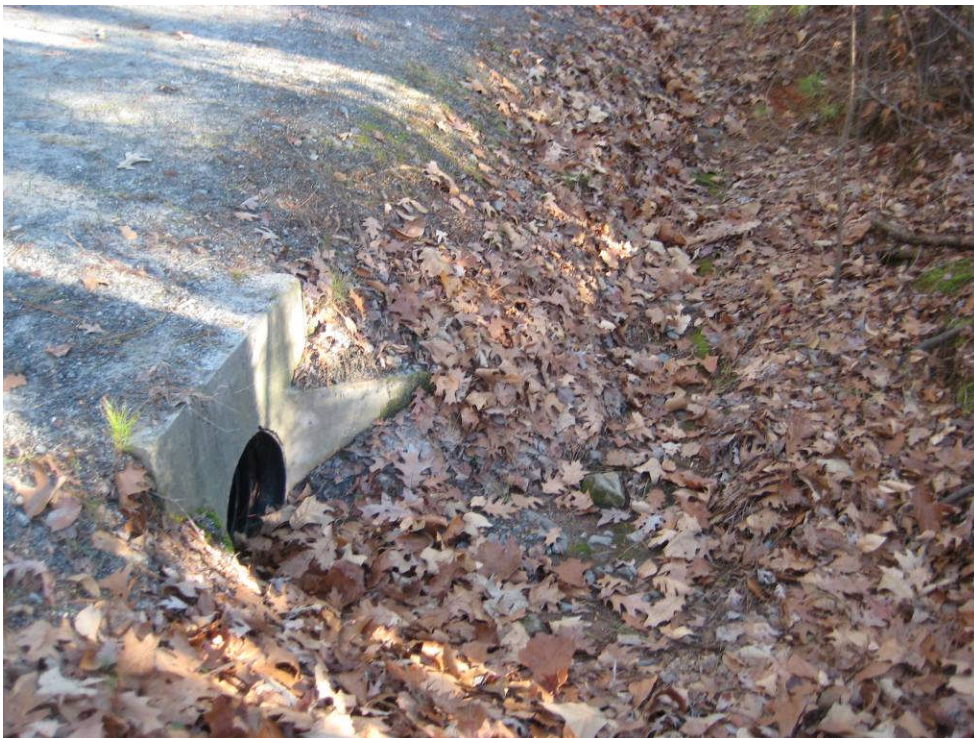
PHOTO F2: upstream face of 18-inch HDPE pipe under trail
