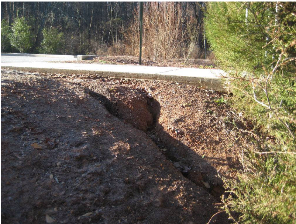
PHOTO – QQ2: rills/ditches in bare soil at northwest edge of Park's Phase III parking lot
