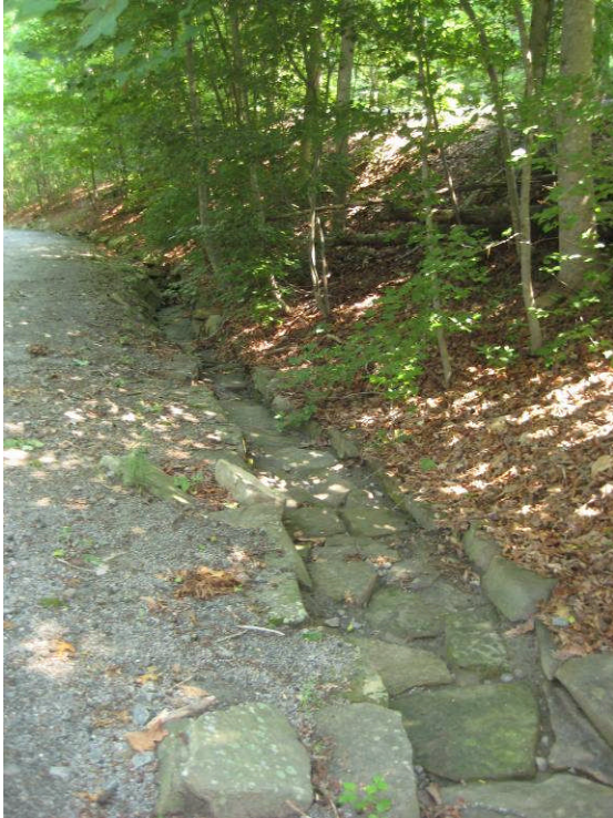
PHOTO E: rock-lined ditch along trail
