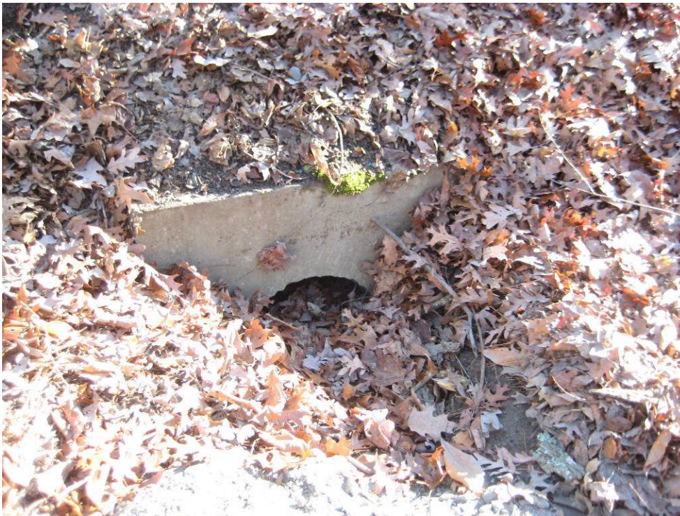
PHOTO E2: downstream face of clogged 18-inch HDPE pipe
