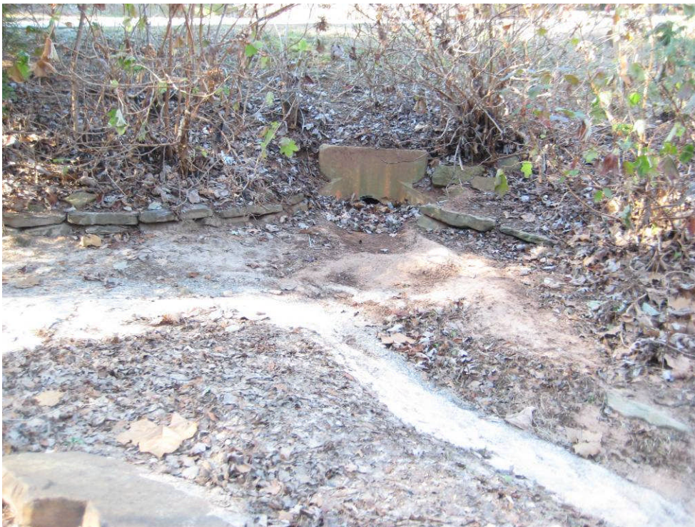
PHOTO – ZZ2: 18-inch HDPE pipe outlet from pipe system that conveys runoff from playground area and the two northern baseball fields (January 2012); same location as Photo ZZ
