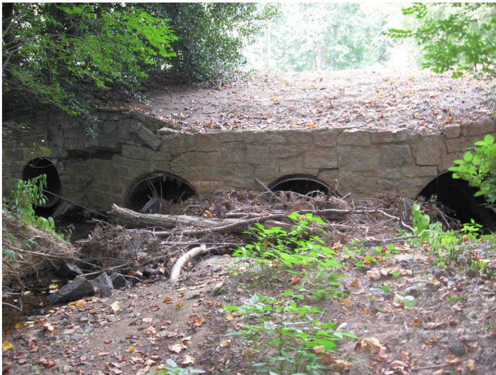
PHOTO – GGG: upstream face of Shirley Bridge Road culvert, triple 54-inch CMPs (taken in August 2011)
