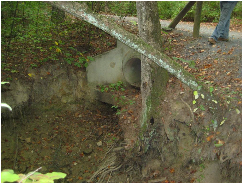
PHOTO J: outfall of 30-inch RCP under trail; erosion undermining headwall
