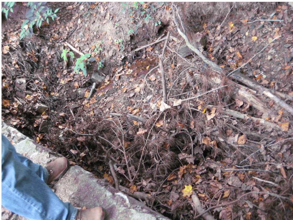
PHOTO – KKK: standing on Shirley Bridge Road culvert, looking at woody debris that has accumulated in channel
