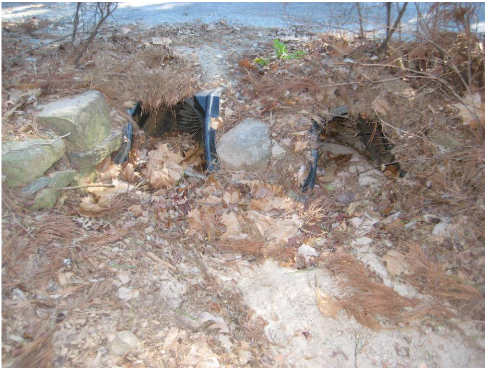
PHOTO – ZZ4: looking at upstream face of double 18-inch HDPE pipes that run under trail to ditch which discharges into pond
