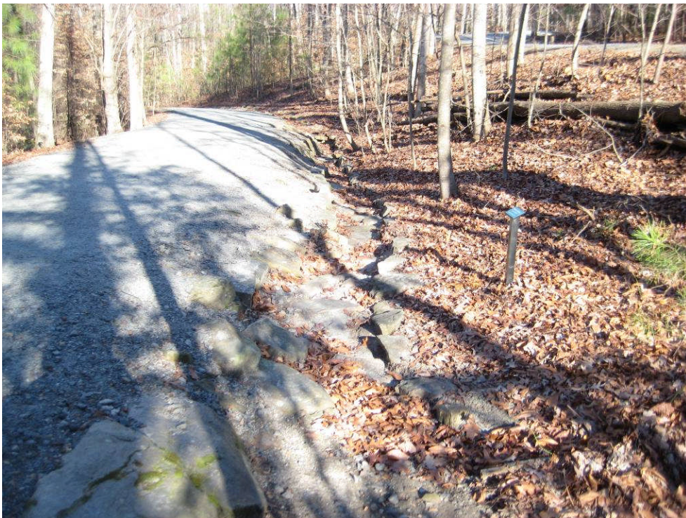
PHOTO D2: at location of pipe outfall from eastern trail, looking downslope at rock-lined ditch
