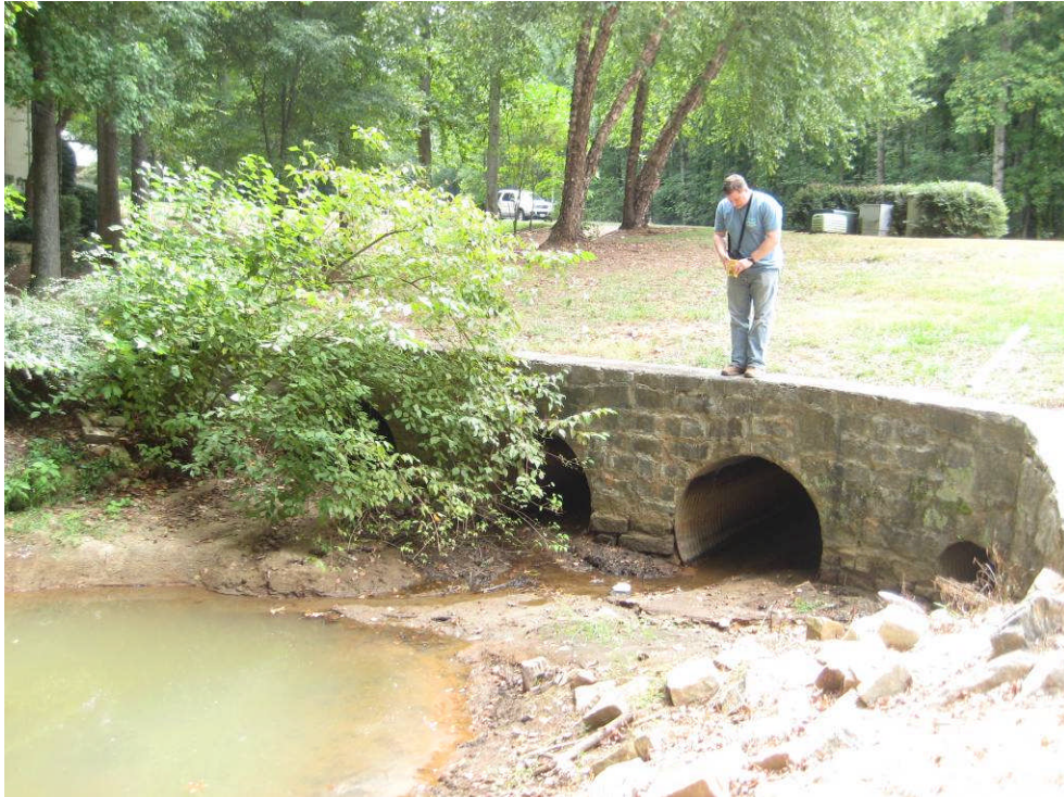
PHOTO – RRR: downstream face of Shirley Bridge Road culvert; sediment has settled out where channel has been widened in the vicinity of the culvert
