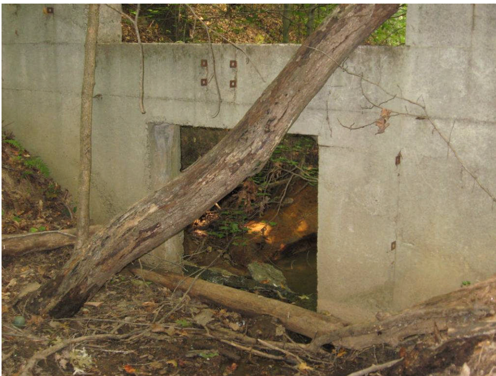
PHOTO HH: upstream face of concrete weir control structure that spans channel
