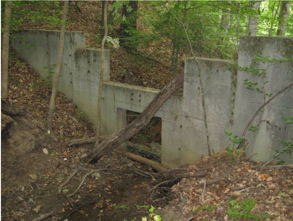
PHOTO JJ: upstream face of concrete weir control structure that spans channel
