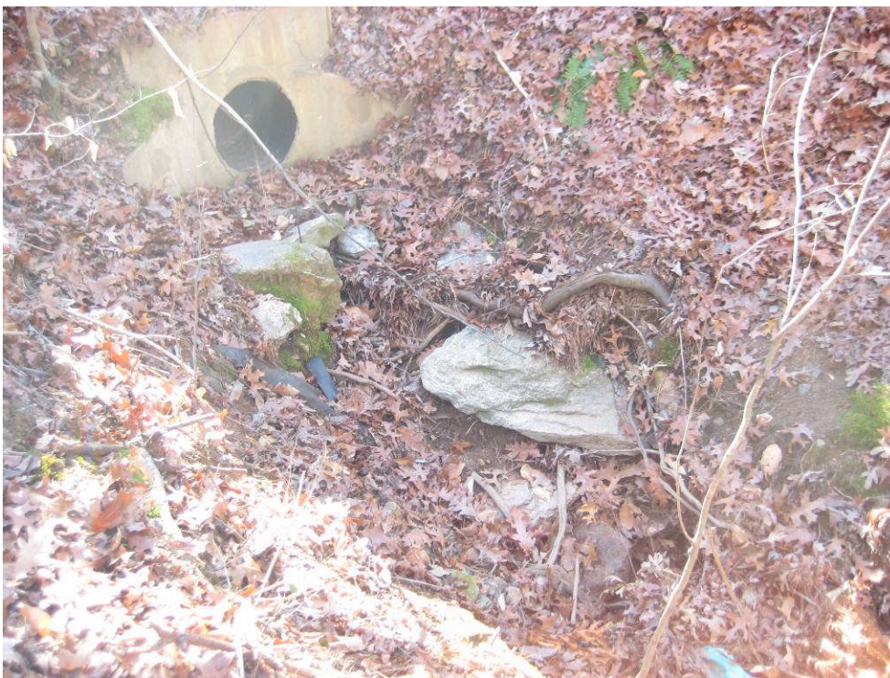
PHOTO C2: erosion at outfall of 18-inch HDPE pipe
