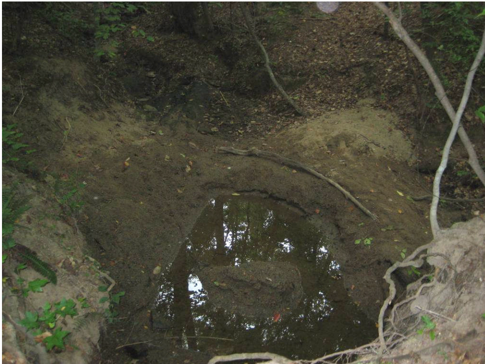
PHOTO Y: scour hole in channel
