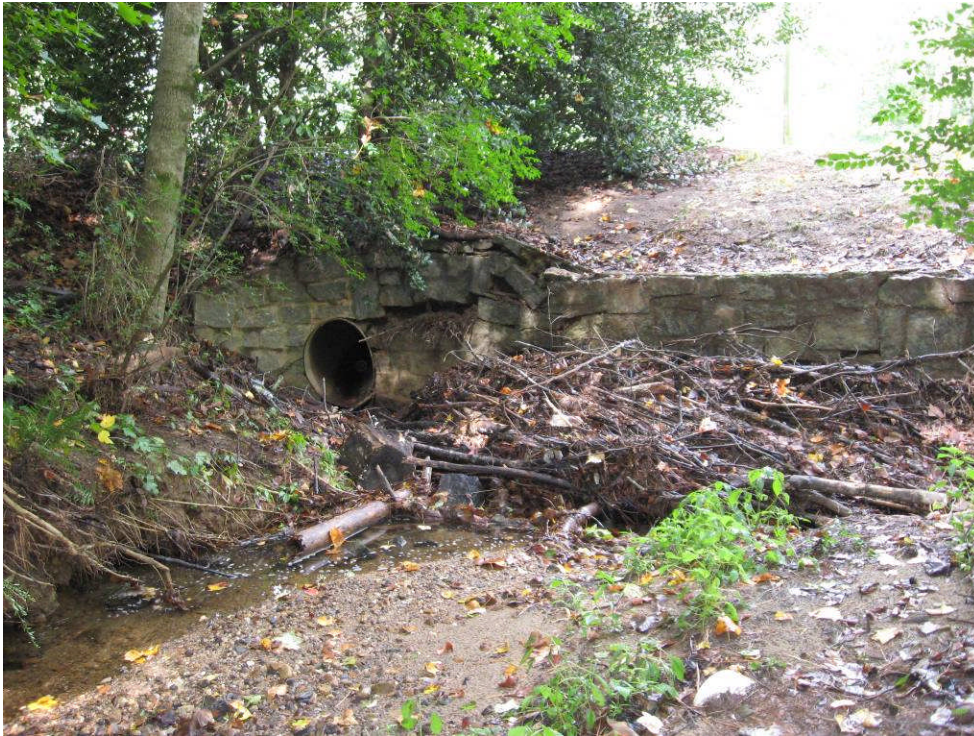
PHOTO – LLL: upstream face of Shirley Bridge Road culvert, triple 54-inch CMPs (taken in October 2011)
