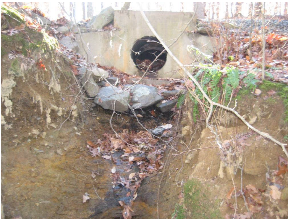
PHOTO T4: standing in stream, looking up at 24-inch HDPE pipe outfall
