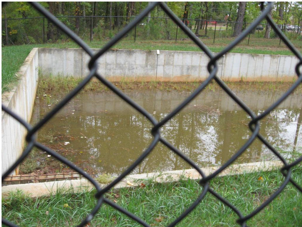
PHOTO – SS: concrete detention pond located behind residential development constructed in 2011; pond is located on private property, just upstream of the park's wet pond; looking south towards homes
