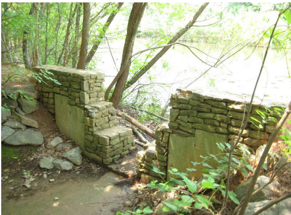
PHOTO – CCC: downstream face of stone weir structure that serves as primary outlet from park pond
