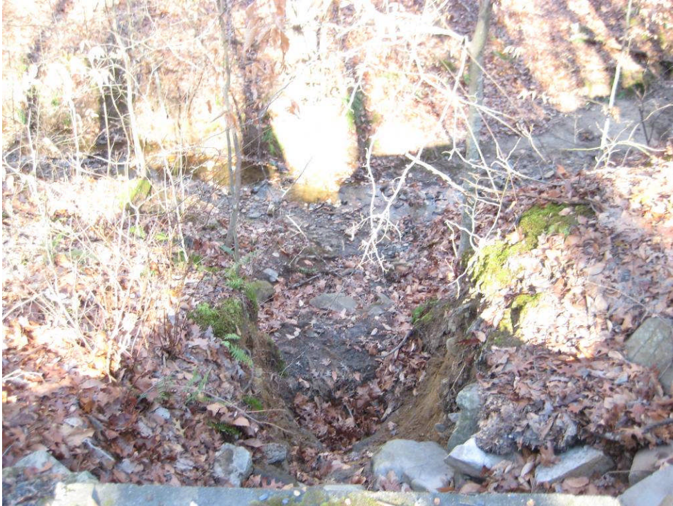
PHOTO T2: standing on headwall of 24-inch HDPE pipe, looking at steep, eroded ditch section between pipe outfall and stream
