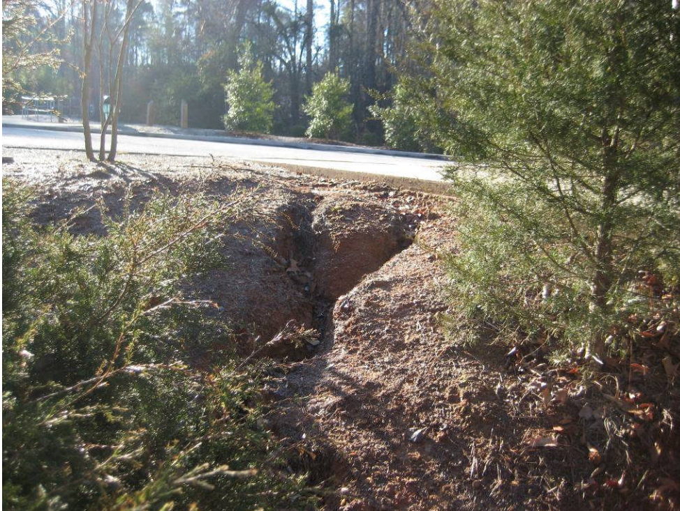
PHOTO – QQ3: rills/ditches in bare soil at northwest edge of Park's Phase III parking lot
