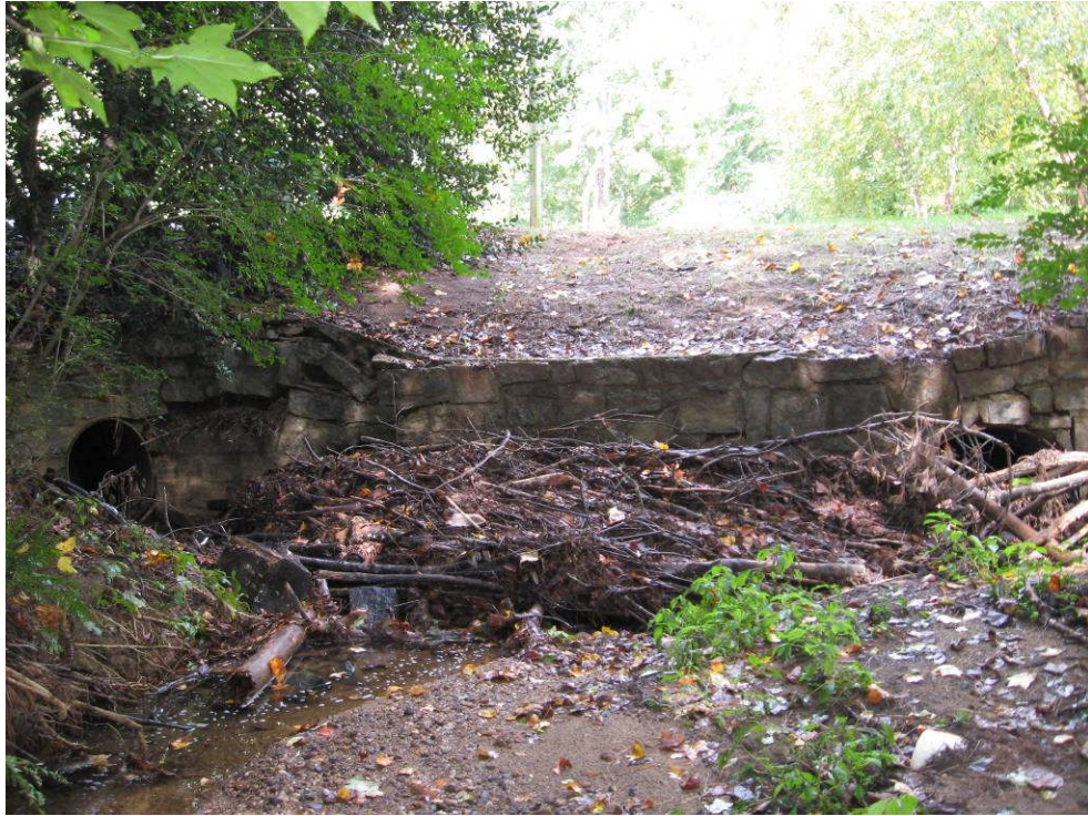
PHOTO – JJJ: upstream face of Shirley Bridge Road culvert, triple 54-inch CMPs (taken in October 2011)
