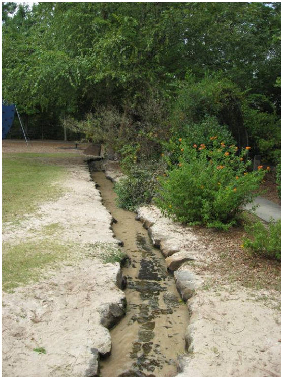
PHOTO – WW: rock channel in playground area, looking downstream (looking southwest) towards outlet, which discharges into pipe system and ultimately into park's wet pond
