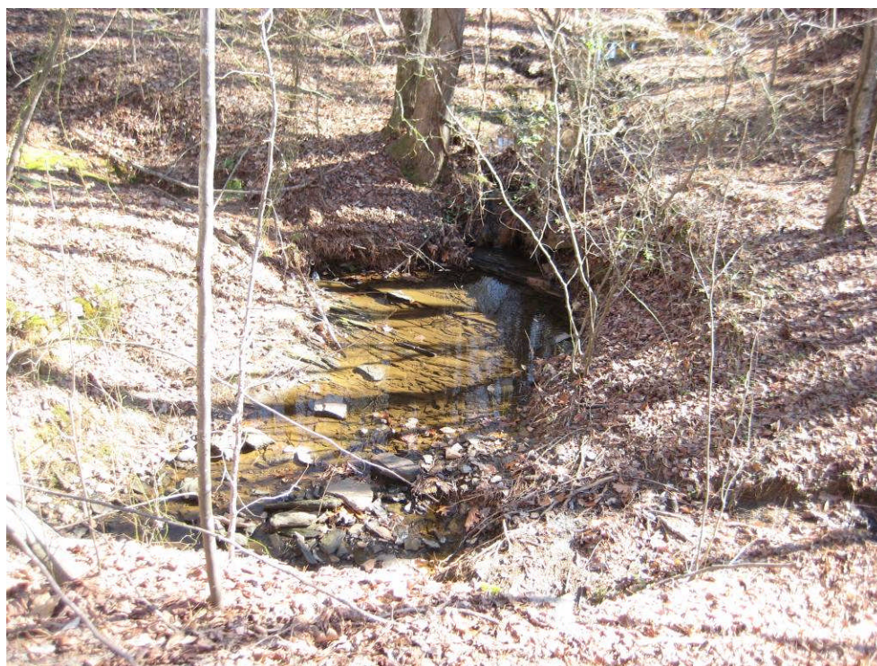
PHOTO – CCC2: localized scour upstream of pipe crossing under trail
