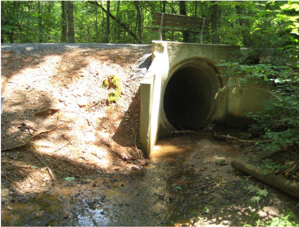
PHOTO R: upstream face of poorly aligned 60-inch RCP
