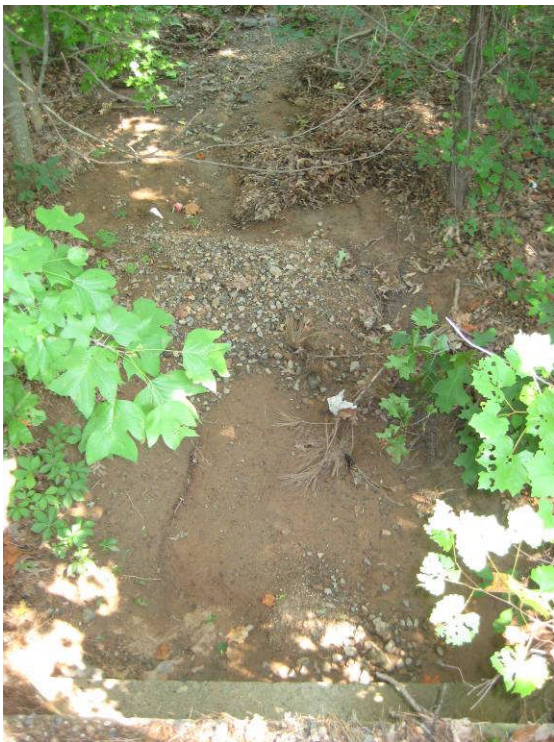
PHOTO C: erosion at outfall of 24-inch RCP
