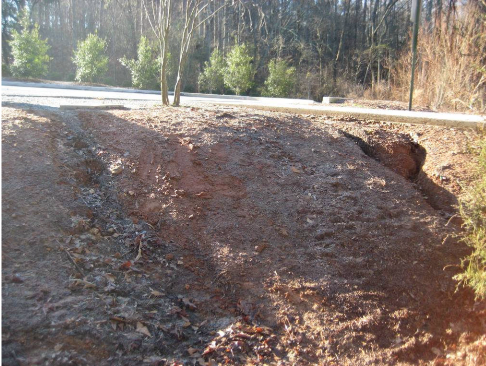
PHOTO – QQ1: rills/ditches in bare soil at northwest edge of Park's Phase III parking lot
