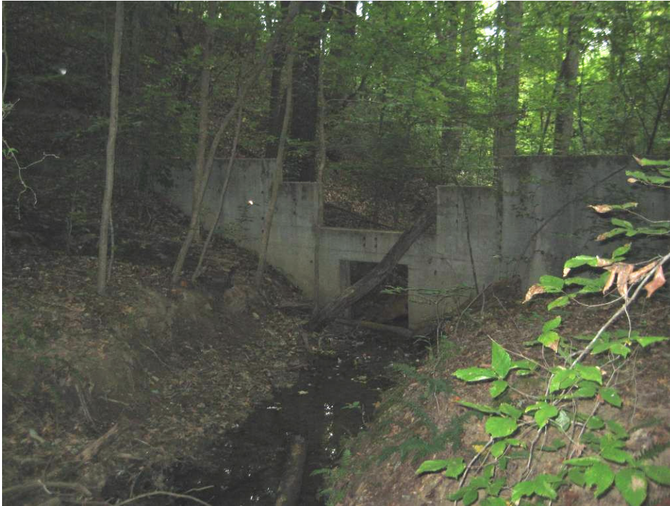
PHOTO HH: upstream face of concrete weir control structure that spans channel
