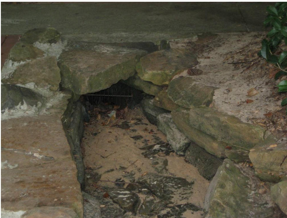
PHOTO – YY: outlet of rock channel in playground area; small metal grate visible under header rock
