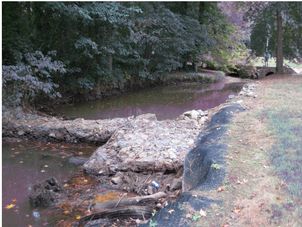
PHOTO – VVV: in-stream gabion structure, located approximately 100 feet downstream of Shirley Bridge Road culvert; looking at downstream aspect of structure (taken in September 2011)
