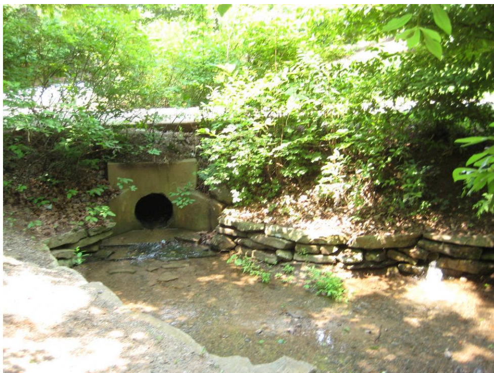
PHOTO – ZZ: 18-inch HDPE pipe outlet from pipe system that conveys runoff from playground area and the two northern baseball fields (June 2011)
