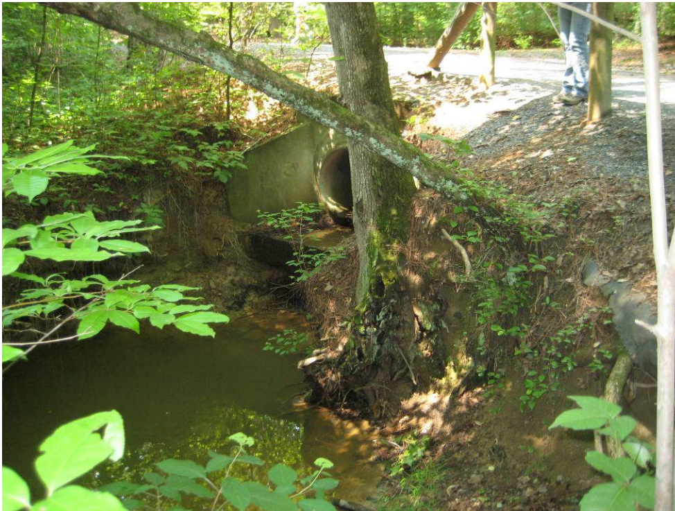
PHOTO L: outfall of 30-inch RCP under trail following rain event; erosion undermining headwall (identical location as Photo J)
