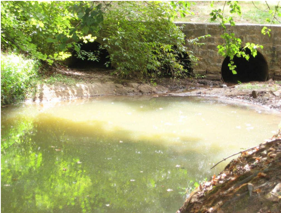
PHOTO – PPP: downstream face of Shirley Bridge Road culvert; sediment has settled out where channel has been widened in the vicinity of the culvert
