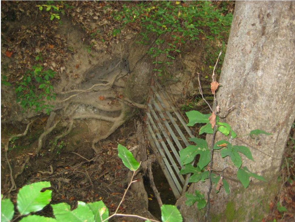
PHOTO LL: metal rack in channel, secured by cables; located at the property limits between the park and the Nottingham Gate subdivision
