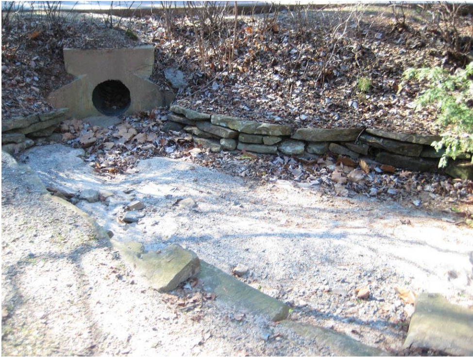
PHOTO – ZZ2: 18-inch HDPE pipe outlet from pipe system that conveys runoff from playground area and the two northern baseball fields (January 2012); same location as Photo ZZ
