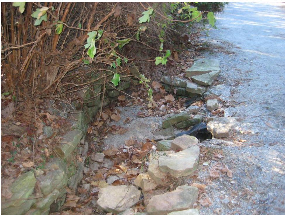
PHOTO – ZZ5: looking upslope at gravel ditch that drains south side of trail; outfall of double 18-inch HDPE pipes, shown in Photo ZZ4, enter ditch from right-hand side of photo; ditch continues downstream directly to pond
