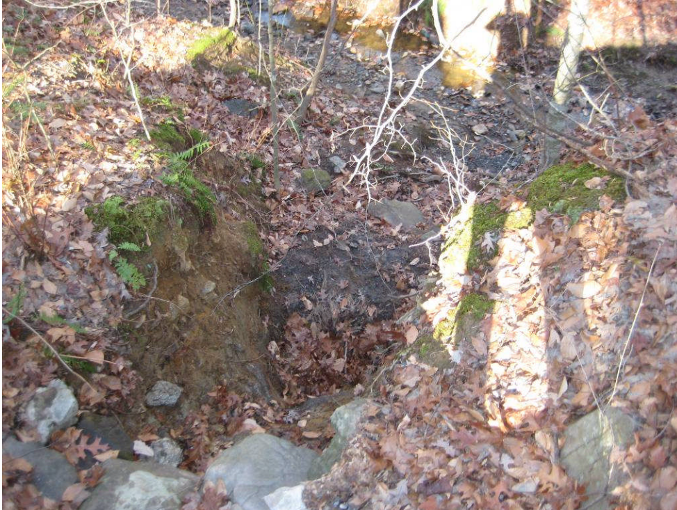
PHOTO T3: standing on headwall of 24-inch HDPE pipe, looking at steep, eroded ditch section between pipe outfall and stream
