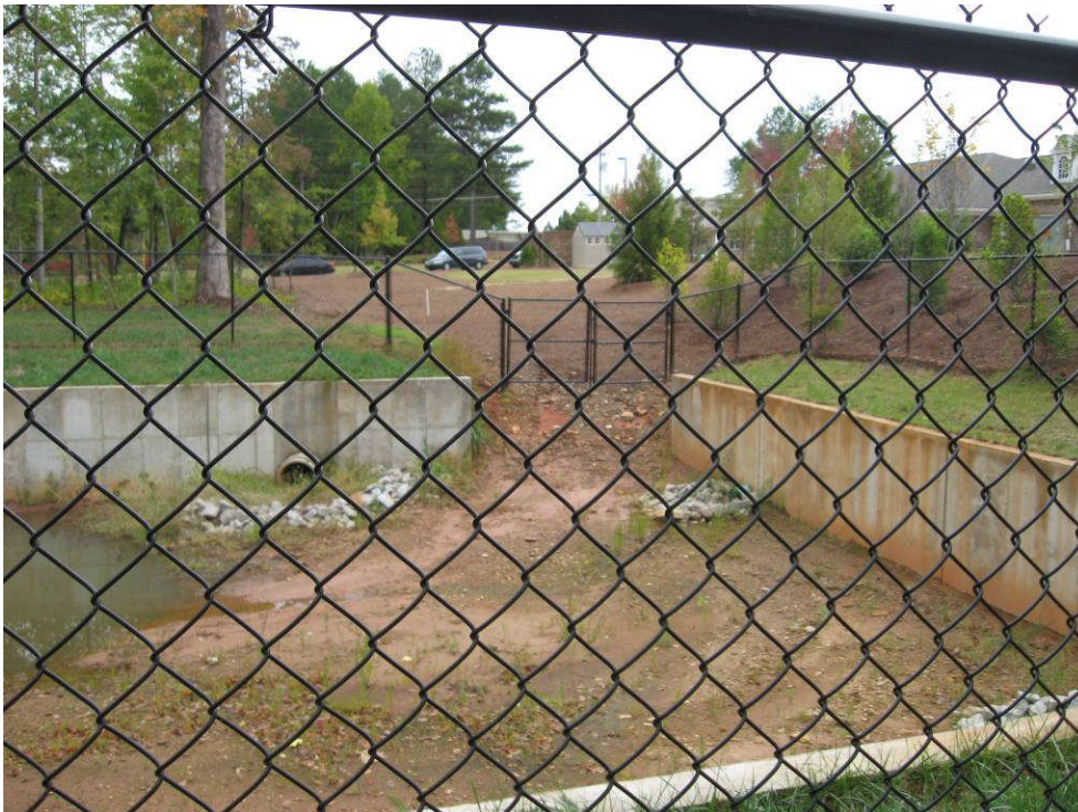
PHOTO – RR: concrete detention pond located behind residential development constructed in 2011; pond is located on private property, just upstream of the park's wet pond
