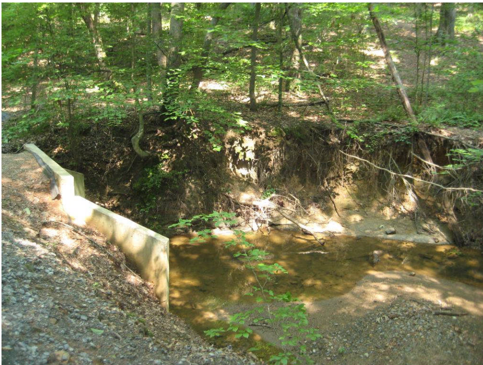
PHOTO S: looking at severely eroded left bank, just downstream of 60-inch RCP
