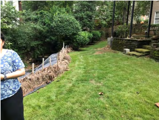
Picture 1: Eroded Streambank
