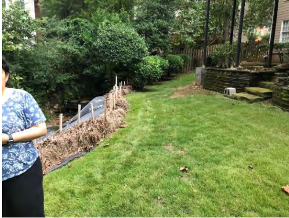
Picture 1: Eroded Streambank
