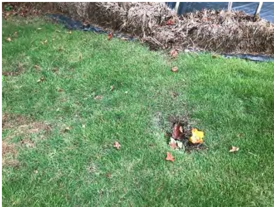
Picture 3: Sinkhole In Backyard
