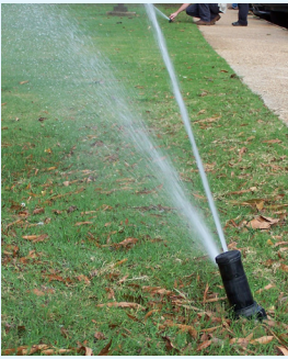
Improperly functioning rotor sprinkler head
