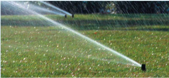
Properly functioning rotor sprinkler head
