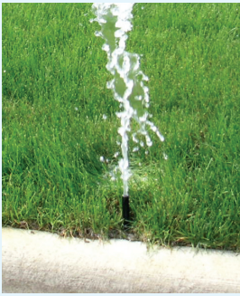
Improperly functioning rotor sprinkler head
