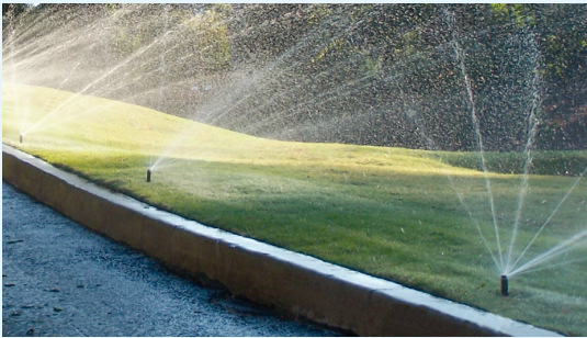
Sprinkler heads are only directed towards grass so that the pavement is not being watered.
