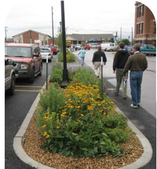
Bioretention areas can be planted to be aesthetically pleasing and look like 'typical' landscape areas.
