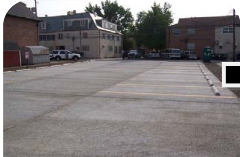
Permeable concrete can be easily integrated into site design and looks similar to traditional concrete.
