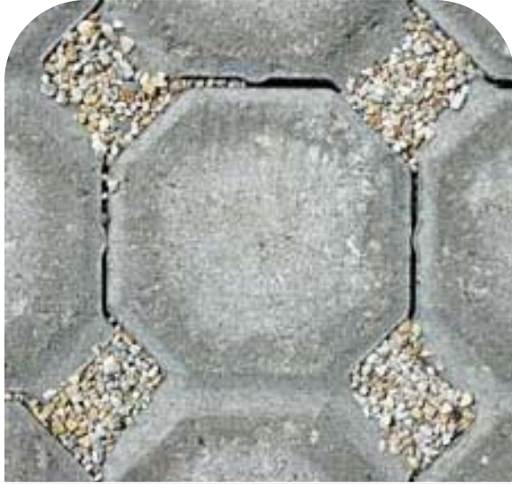
Fine aggregate allows water to infiltrate in gaps between interlocking pavers. Pavers are well-suited to plazas, patios, and small parking areas where aesthetics are important. Photo courtesy of www.nrdc.org .
