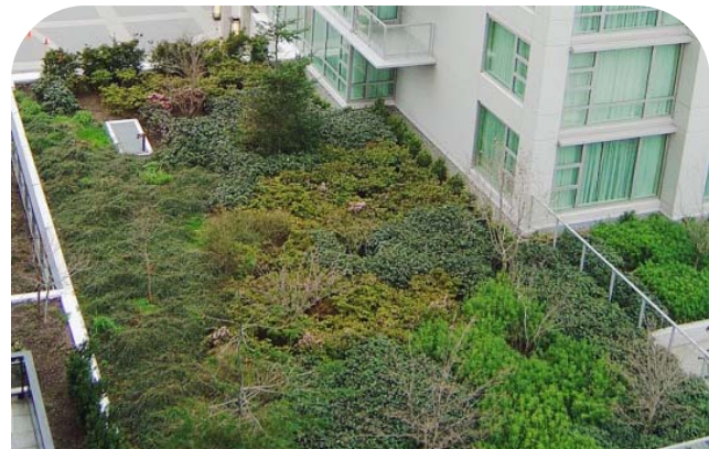
Intensive Green Roof Example. Intensive green roofs are usually accessible to others (besides maintenance) and allow for great plant diversity.
