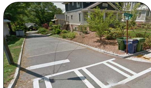
Permeable concrete used in a roadway application. Feder Avenue, Atlanta
