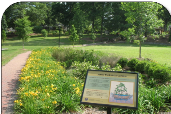
A healthy and properly maintained bioretention area.
