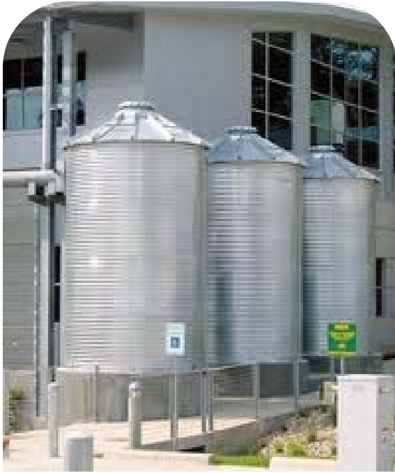
Placement of storage tanks higher than areas where water will be reused may reduce or eliminate pumping needs. Photo courtesy of www.winebusiness.com .
