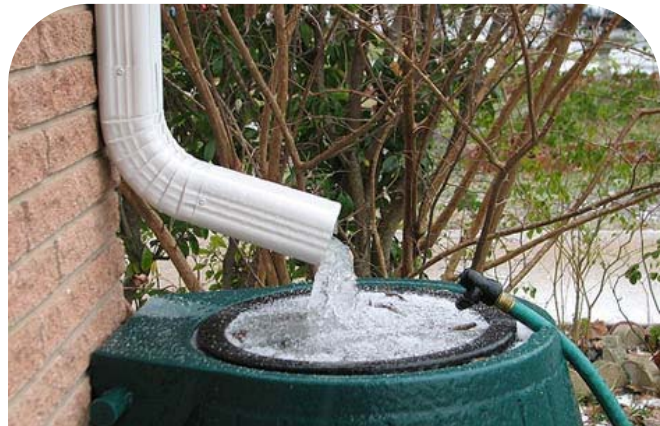
Screens are an acceptable form of pretreatment for rainwater harvesting systems. Photo courtesy of www.treehugger.com .
