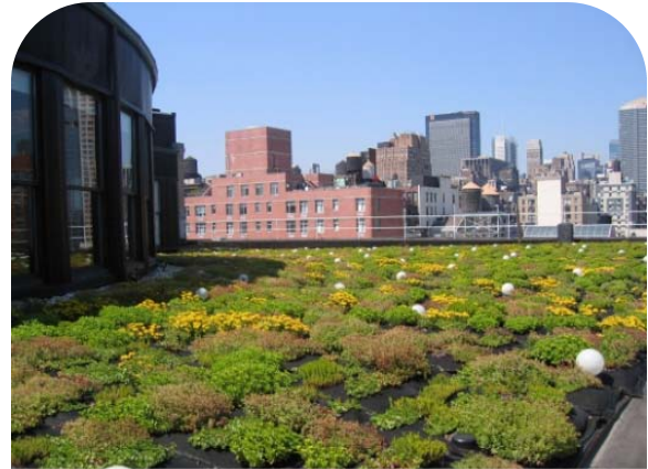
Green Roof with Sedum Mix
