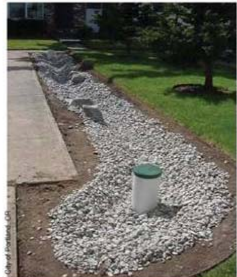
An Infiltration Trench can fit into tight spaces that are typical of small commercial sites. Photo courtesy of: http://www.portlandoregon.gov/bes/article/202883
