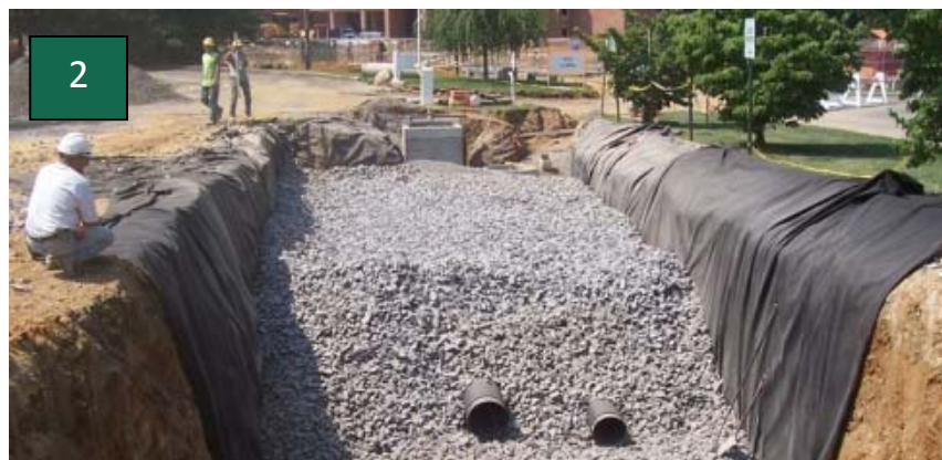
Figures depicting: (1) a subsurface infiltration facility cross section, (2) a facility during construction, and (3) a facility after construction is complete. Photos courtesy of: http://www.csc.temple.edu/t-vssi/BMPSurvey/delaware_countycc.htm and http://www.esf.edu/ere/endreny/GI/Calculator/InfiltrationIntro.html
