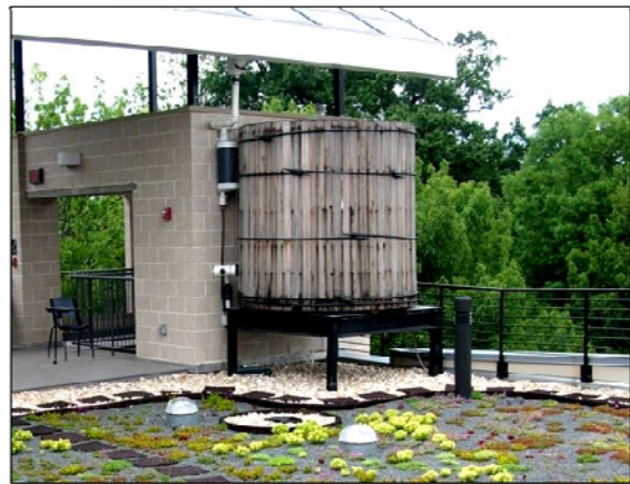
Cistern used in conjunction with a green roof. Southface, Atlanta, Georgia.
