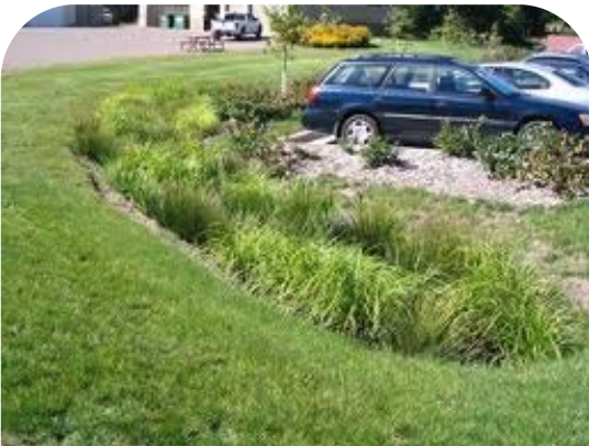
A healthy and properly maintained bioswale. Photo courtesy of www.rwmwd.org .
