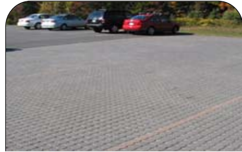
Permeable paver parking stalls add variety to parking lot landscape. English Park, Atlanta
