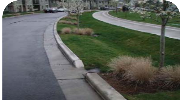
Curb cuts used to drain water from roadway to bioswale. Photo courtesy of www.indygov.org/eGov/City/DPW/SustainIndy/WaterLand/Documents/Final.pdf
