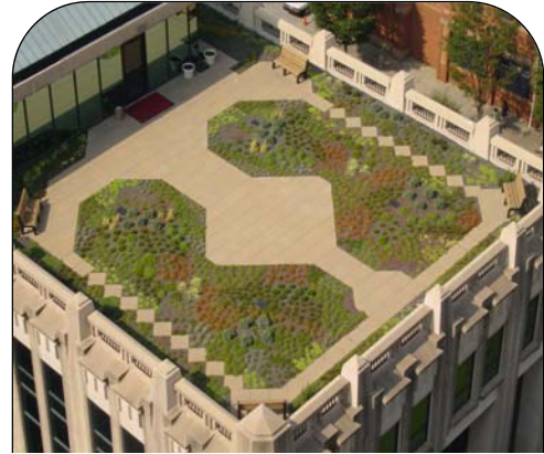
City Hall Green Roof. Atlanta, Georgia
