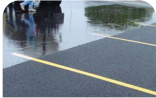
Comparison of permeable asphalt (left) with traditional asphalt surface (right) during a storm event. Photo courtesy of www.wolfpaving.com
