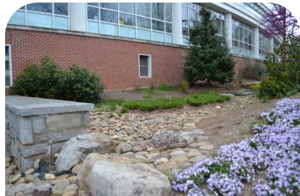
Terraced bioswale accepts runoff from roof drains. Grade control structures allow infiltration Klaus Building - Georgia Tech – Atlanta, Georgia
