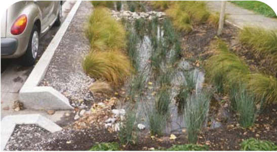
Curb cut entrance to bioswale. Photo courtesy of www.americanforests.org .
