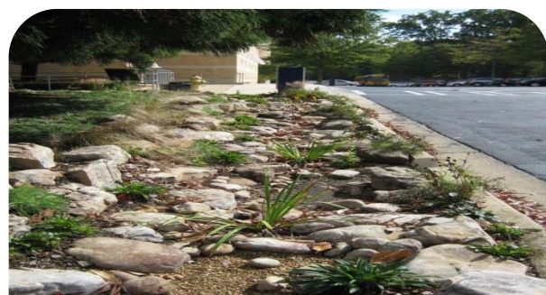
Bioswales can function as a substitute for parking lot curb and gutter systems.
