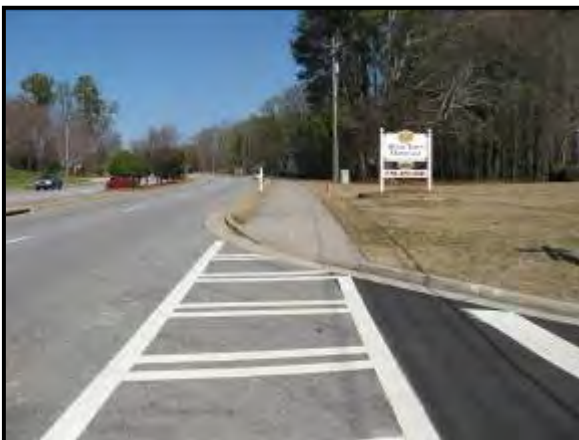
Figure 14 Sidewalk-to-Ramp width inconsistency along Haynes Bridge Road
