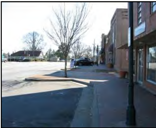
Figure 8 Example of Curb Extension along South Main Street
